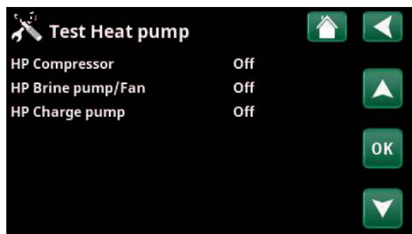
Menu: "Advanced/Service/ Function test/Heat pump".
